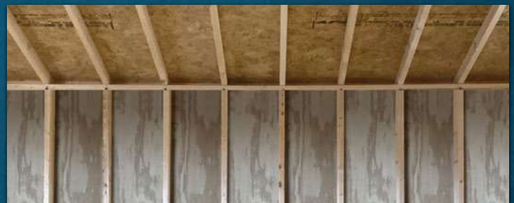
16" ON CENTER STUDS & TRUSSES (TREATED ONLY) | F2
