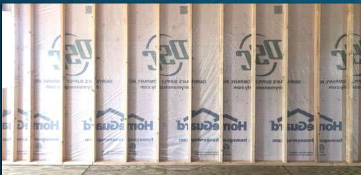
HOUSE WRAP VAPOR BARRIER | P1
